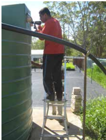
Kanna and Ranjan putting the overflows into one of the new tanks.
