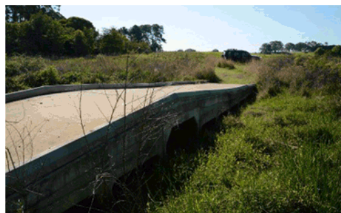
Wetland Outlet Structure
